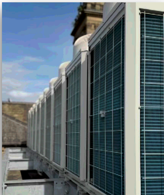
Air source heat pumps at Morley Town Hall installed with Public Sector Decarbonisation Scheme money.
