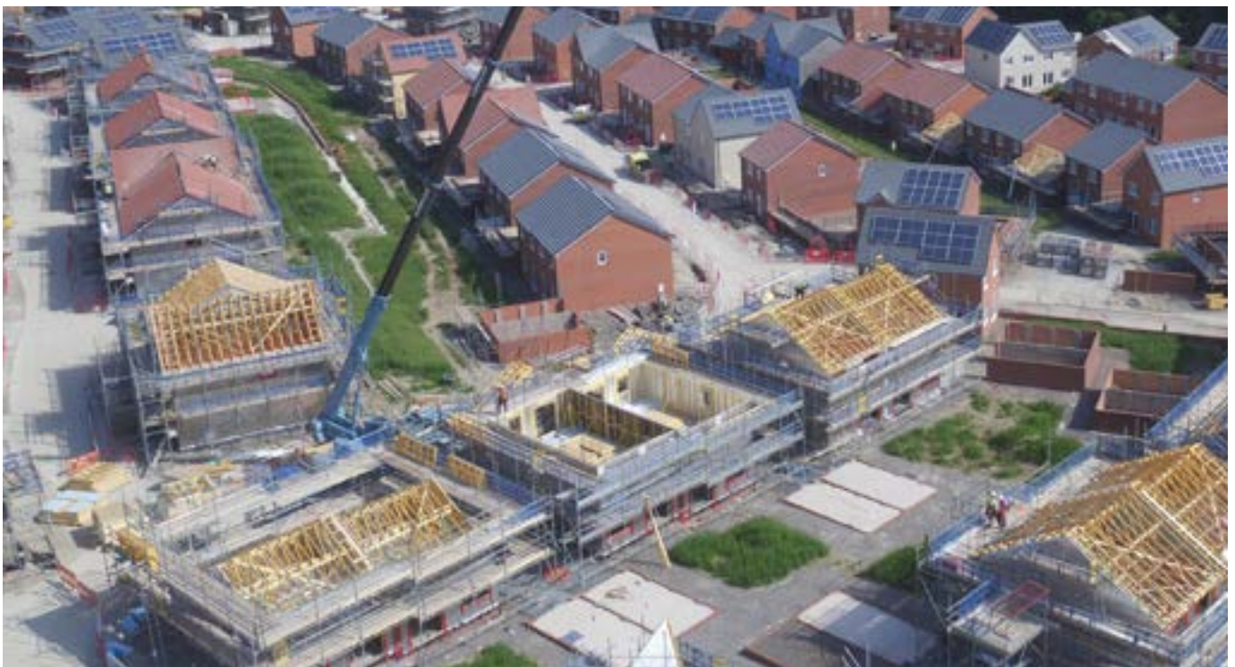
New homes being built on Defence development land at Bulford, Wiltshire
