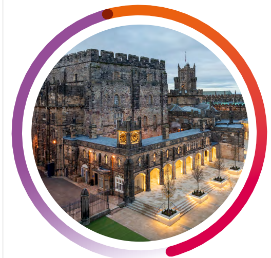
Lancaster Castle, designed by architects BDP.
