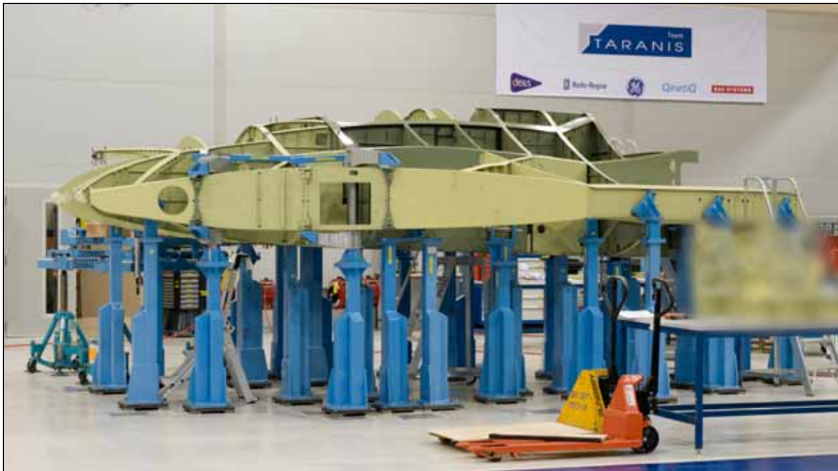
Taranis Under Construction
