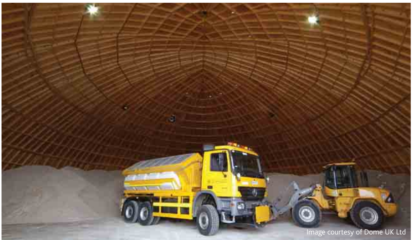
Figure 5.2: Loading inside a salt barn
