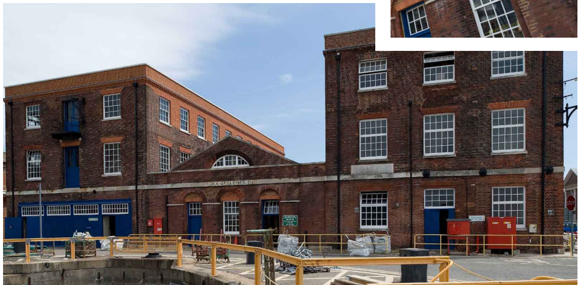
Block Mills, Portsmouth Naval Base, a scheduled monument and Grade I listed
