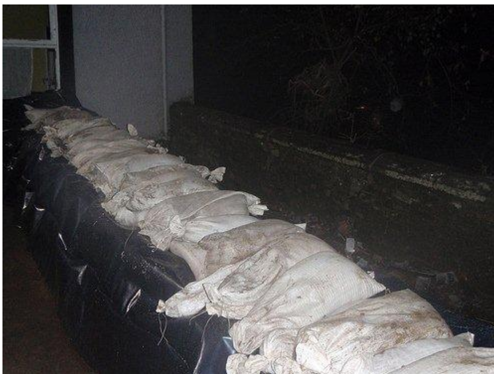
Picture 12: Environment Agency staff worked to shore up flood defences in Cockermouth during the flooding in November 2009
