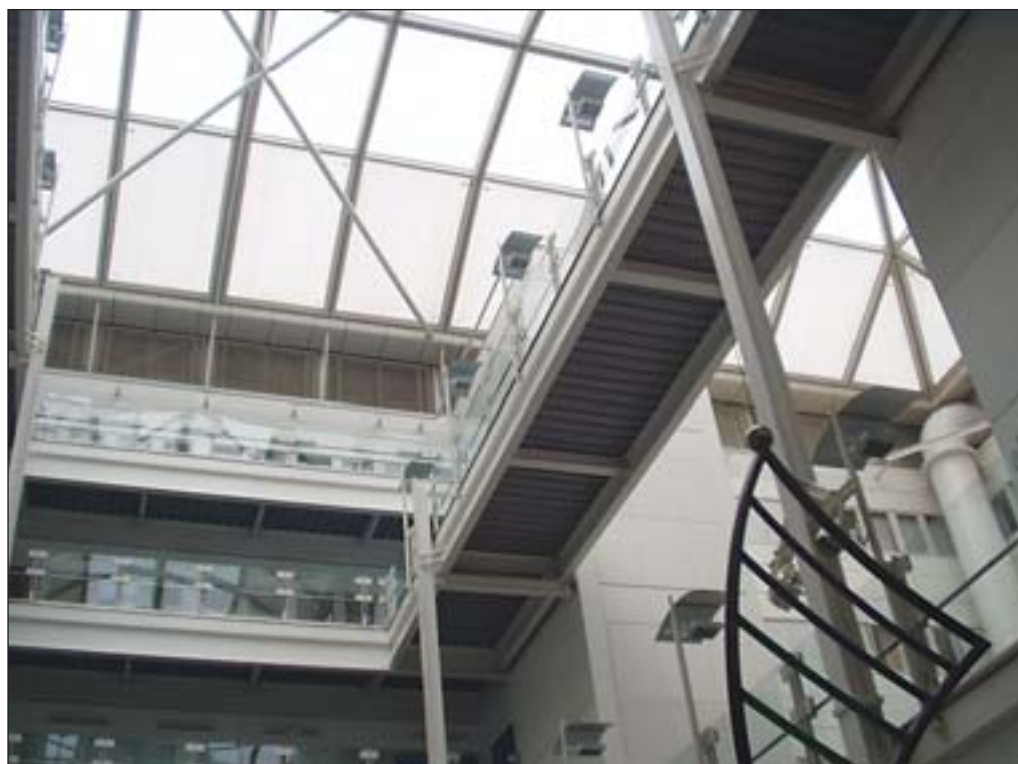
An internal view of the atrium at Chelsea and Westminster Hospital, affording good levels of natural light to the hospital interior (see box "Atria" in Chapter 4 for further guidance on the use of atria for saving energy)
