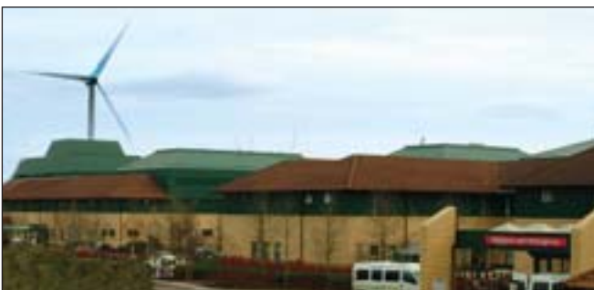
The 660 kW wind turbine at Antrim Area Hospital was the first to be installed on a hospital site in Northern Ireland. The scheme is on track to save £90,000 in its first year of operation.
