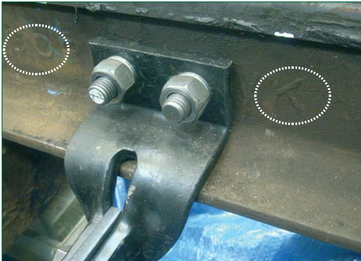
Figure 10: Rail branding on right-hand switch rail (Note: a new bracket has been added for testing purposes)
