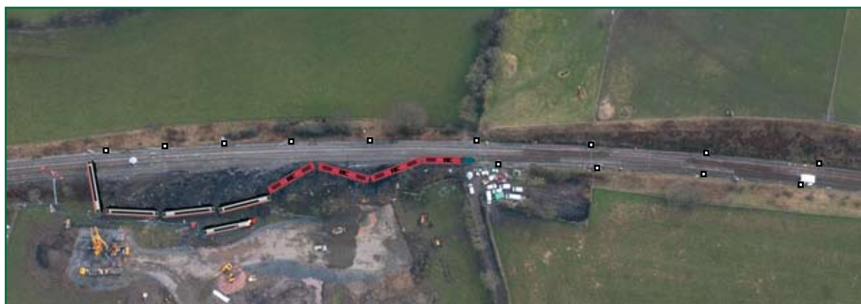
Figure 36: Final location of the vehicles from train 1S83 after the derailment
