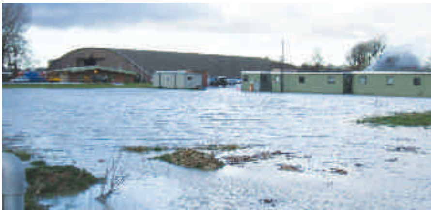
Flooding, RAF Brize Norton
