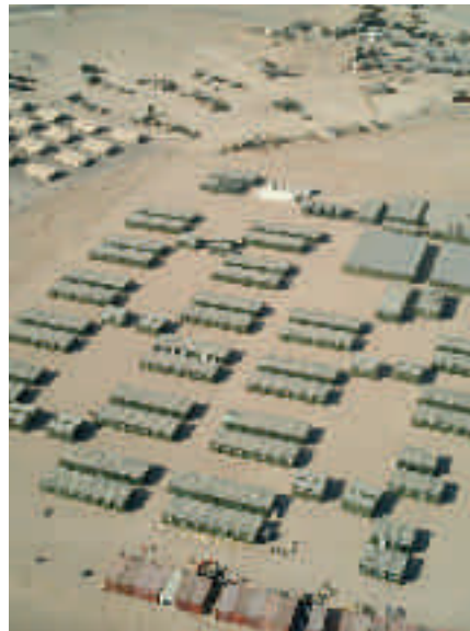
Gundulph, Temporary Field Accommodation, Iraq
