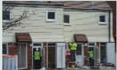
Upgrading of SFA, Dale Barracks
