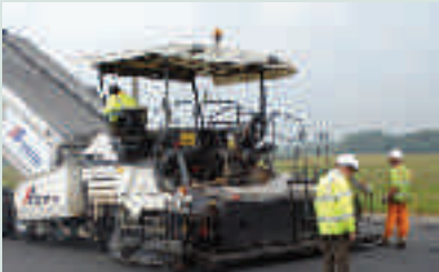
Final coat of Marshall Asphalt, RAF Linton-on-Ouse
