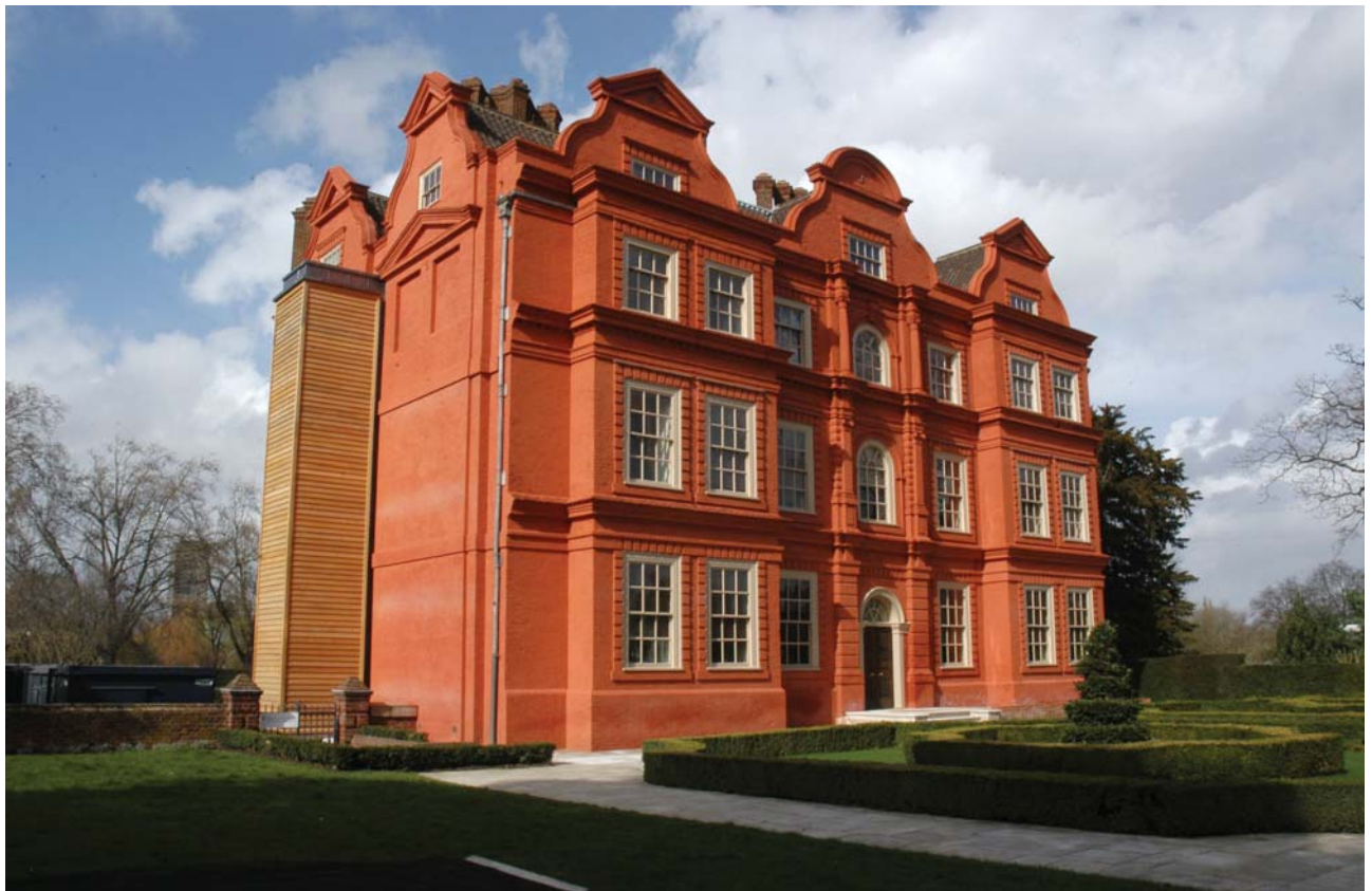
Kew Palace exterior, showing the new timber-clad lift shaft. The brickwork is painted with limewash coloured with brick dust in imitation of the eighteenth-century decorative scheme.
