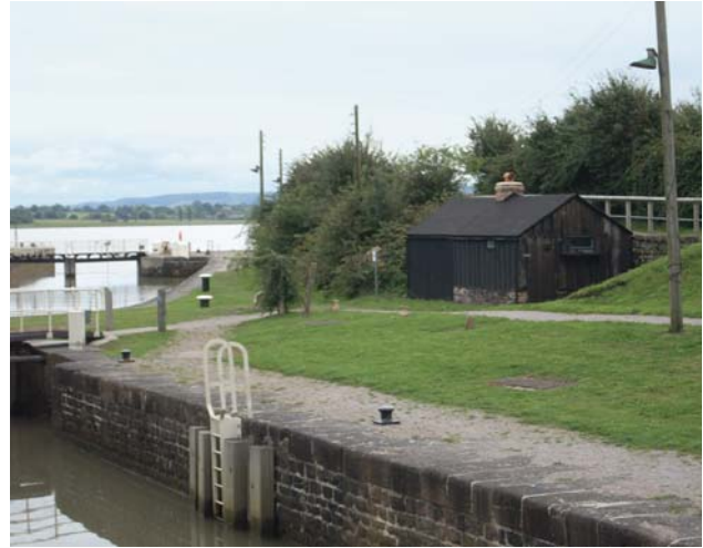
View from lock chamber between inner and outer harbours (foreground), towards the outer harbour. Generator shed to the right.
