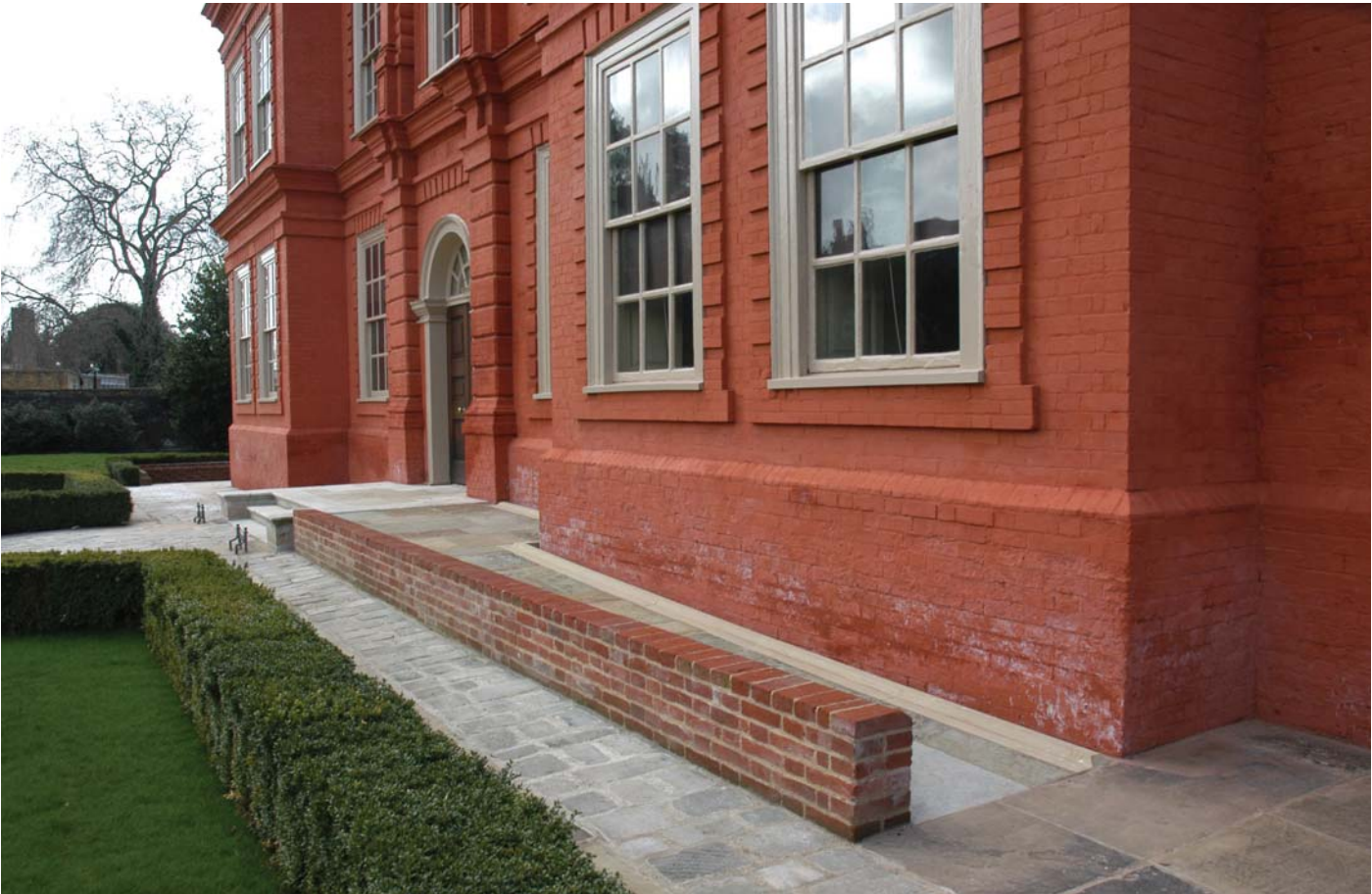
The new access slope outside the front entrance to Kew Palace. The slope is hidden from long views of the palace by the formal box hedging.
