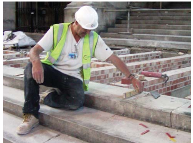
Relaying the treads
