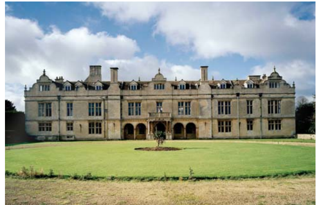
East range in 2004, prior to repair
