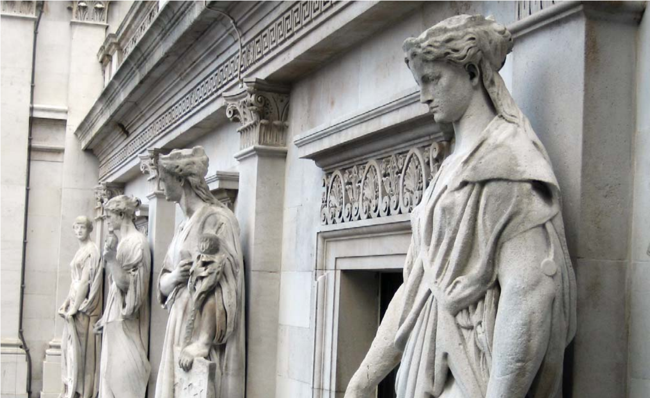
East elevation statues after cleaning and repair
