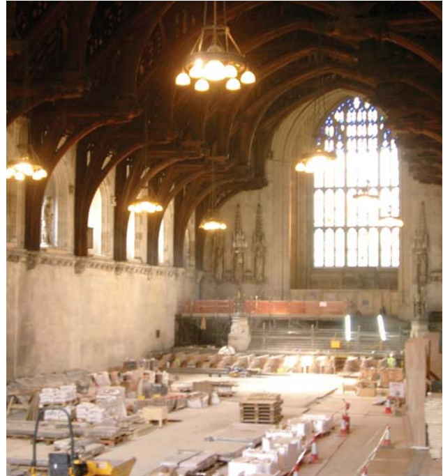
Westminster Hall during the works
