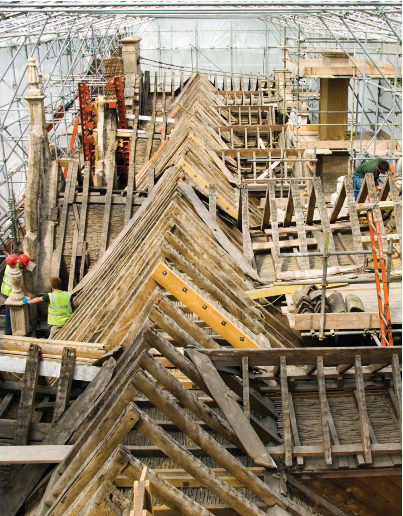
Roof repairs in progress, 2006
