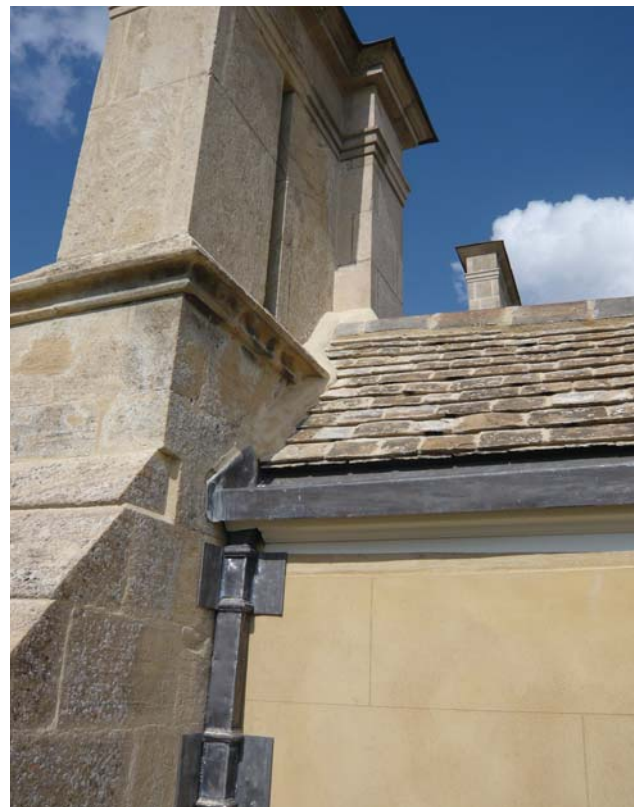
Detail of completed roof repairs, 2007
