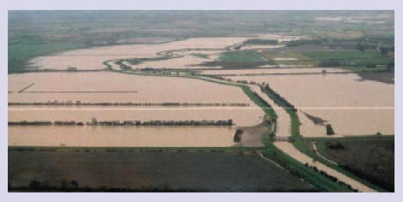
Till washland in flood – the embankment and control sluice (foreground) hold back the water from passing downstream to Lincoln.
