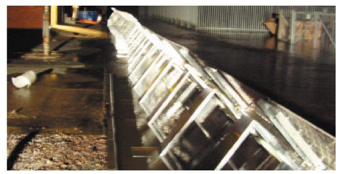
Temporary defences set up to protect Walham electricity switching station – preventing around 450,000 domestic and commercial customers losing power
