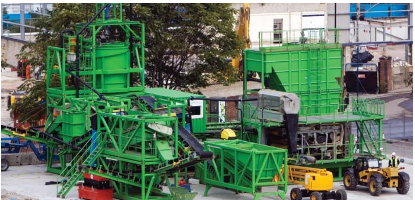
Soil washing machine working on the Olympic Park site
