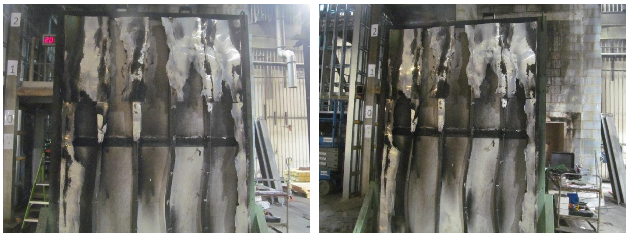
Figure D57 – Post fire observations
