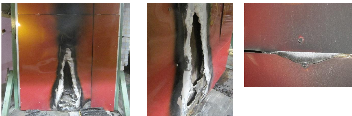
Figure D32 – Post fire observations
