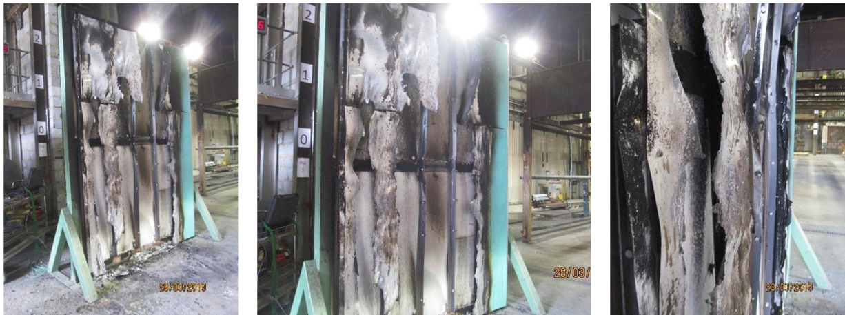
Figure D37 – Post fire observations
