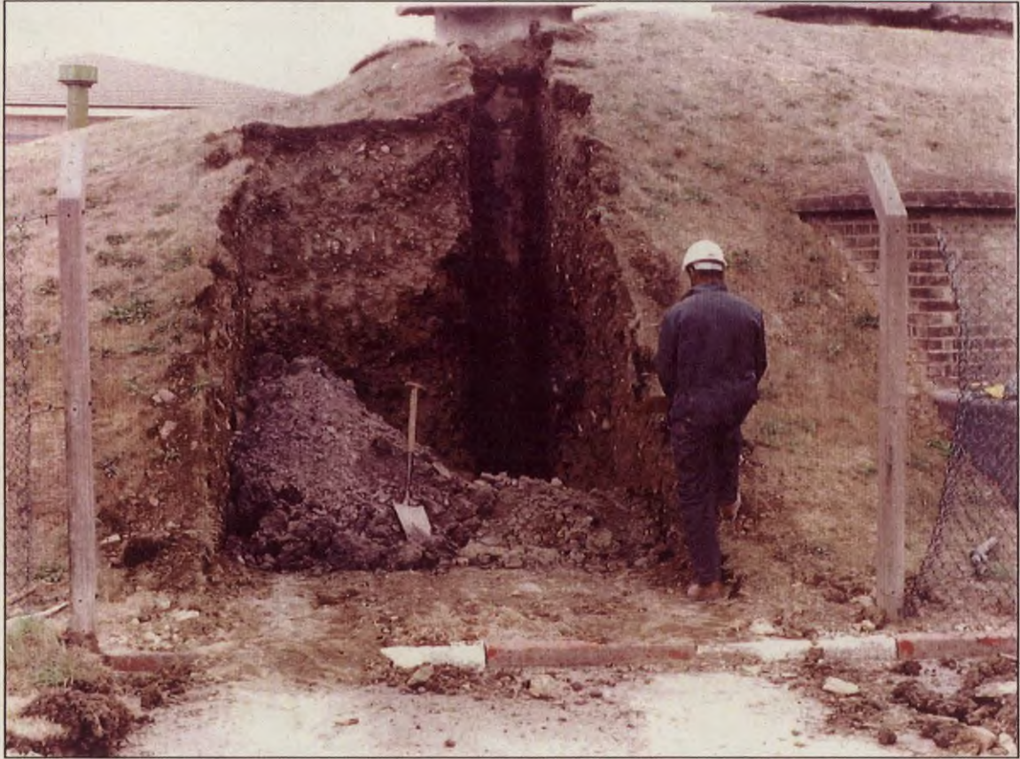
Figure 26. Removal of BFI 1 – trial pit showing concrete ring structure extending vertically.
