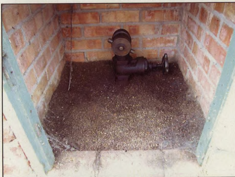
Figure 49. Fill point for the fuel tank at Scampton Primary School, located in the RAF Scampton visitor's car park.
