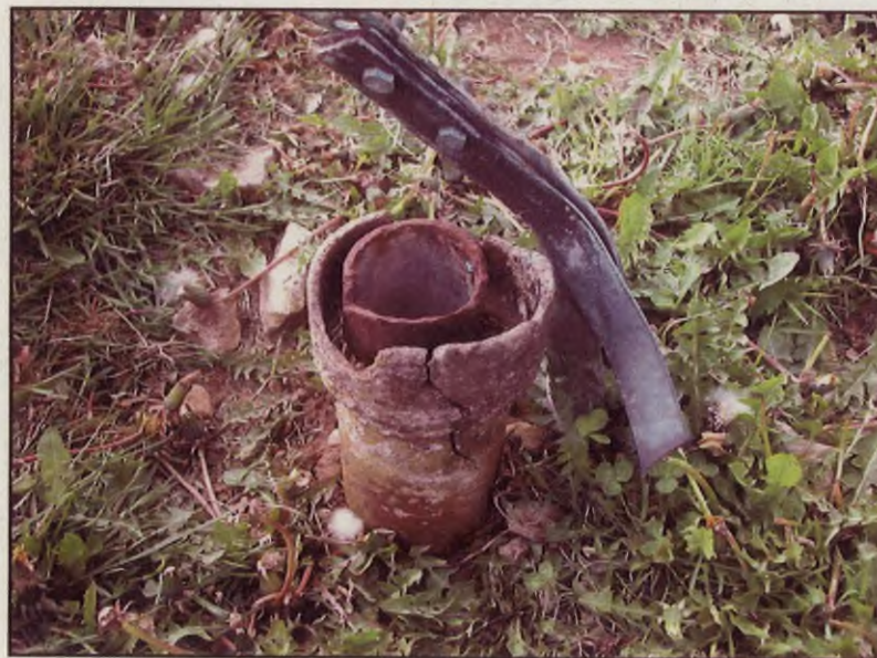
Figure 24. Asbestos type material forming a sleeve around a vent pipe.
