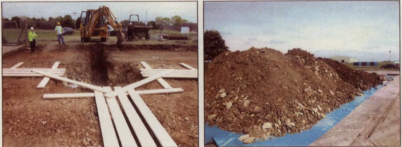
Figure 39. (left) Trial pits dug to assess extent of contamination and (right), resultant spoil.
