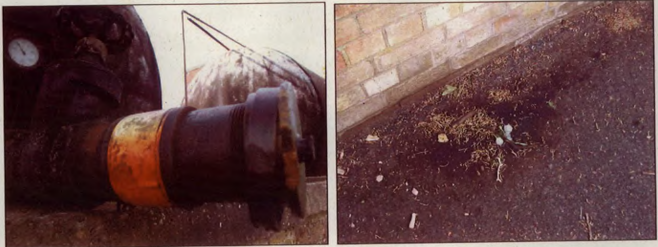
Figure 43. Diesel found dripping from a Standby Set House (Bldg No 157) tank fill point (left) onto the tarmac road (right).
