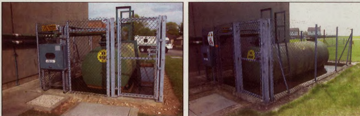
Figure 47. Water filled bunds at Uniter NUB 1 & 2 (Bldg Nos 601 and 602).
