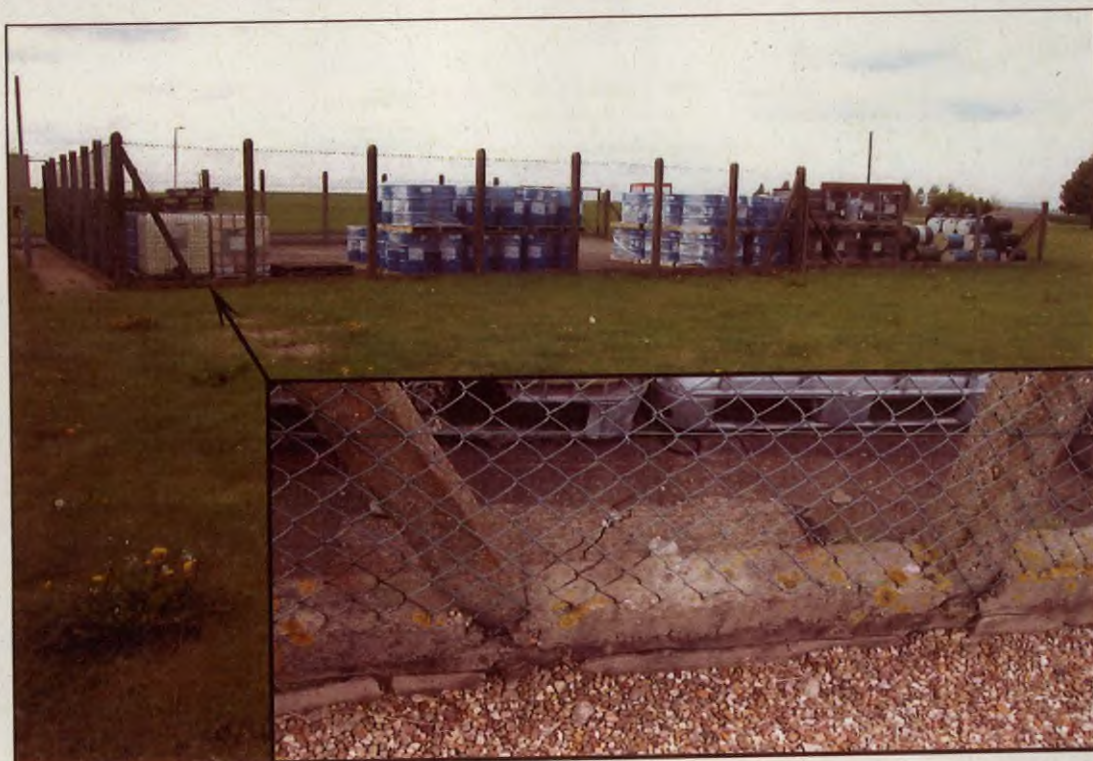
Figure 41. Waste oil compound (Bldg No 498) showing cracked bunding around the edge and on the compounds concrete base.
