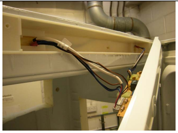
Photo 7 Controller – cable entry via sandwich panel
