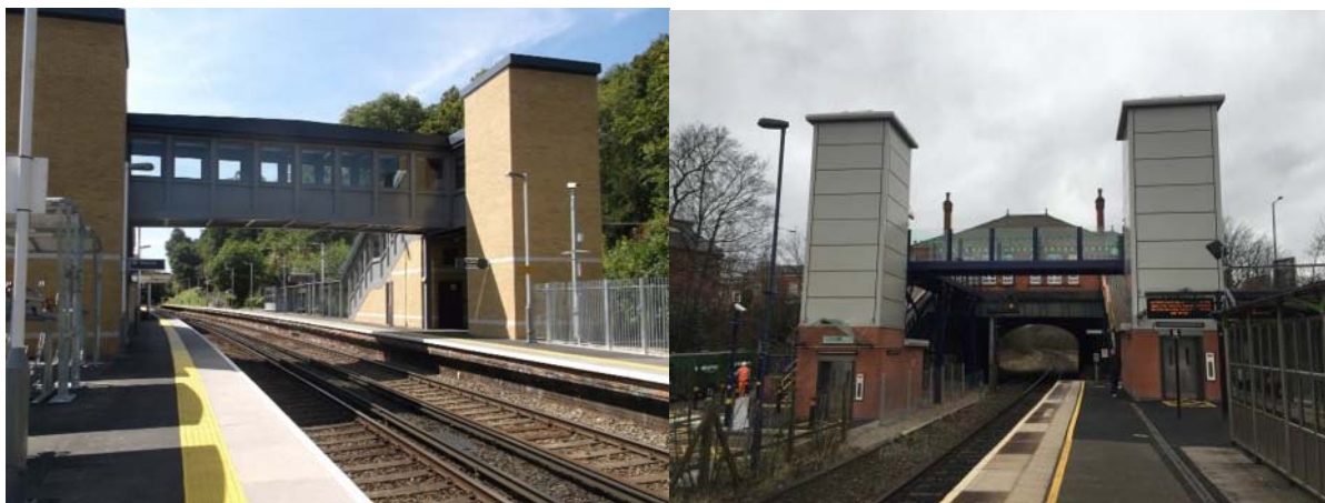
Image 2: Access for All improvements at Godalming and Acocks Green railway stations
