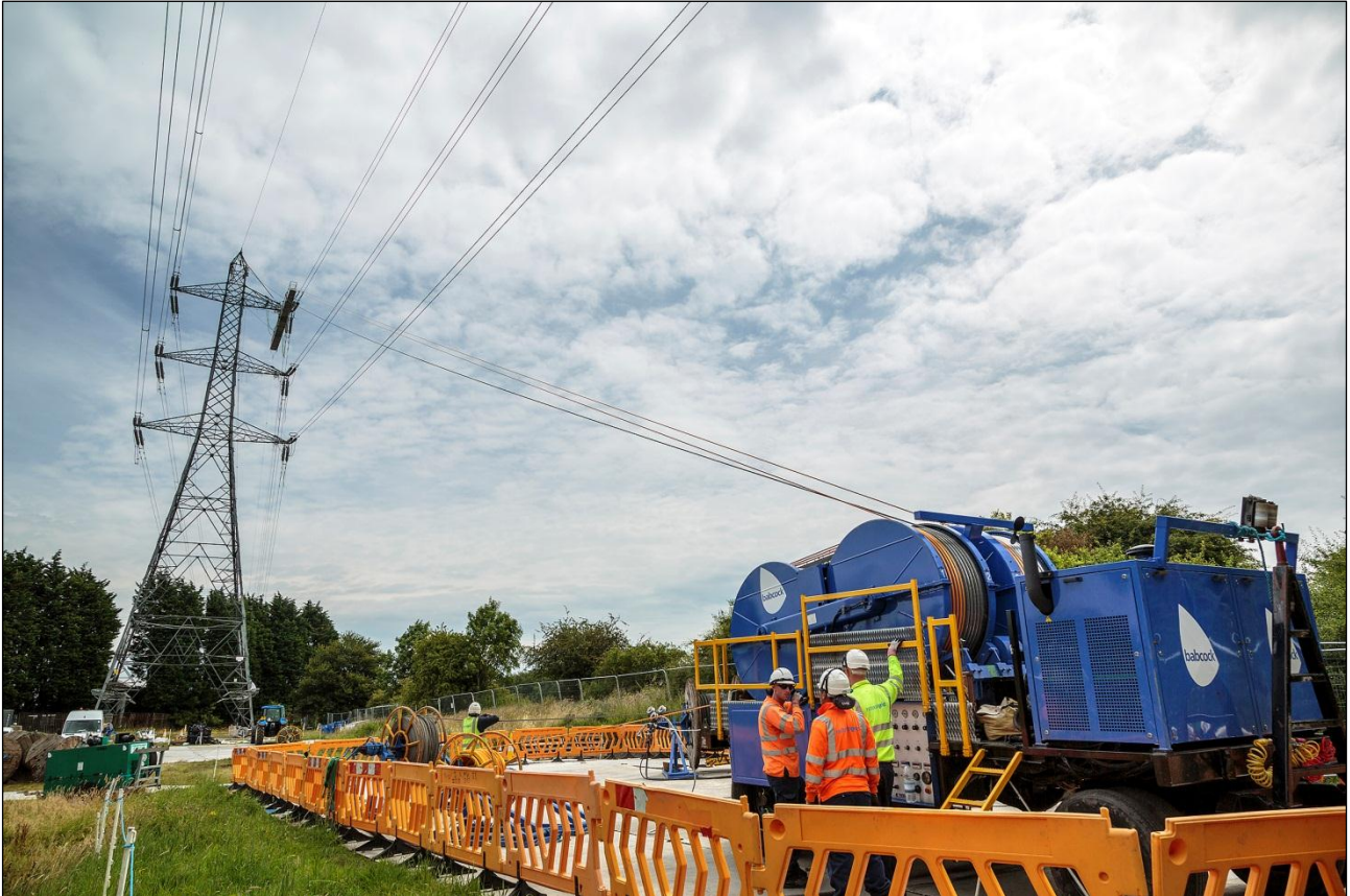
Figure 3: Typical winching site
