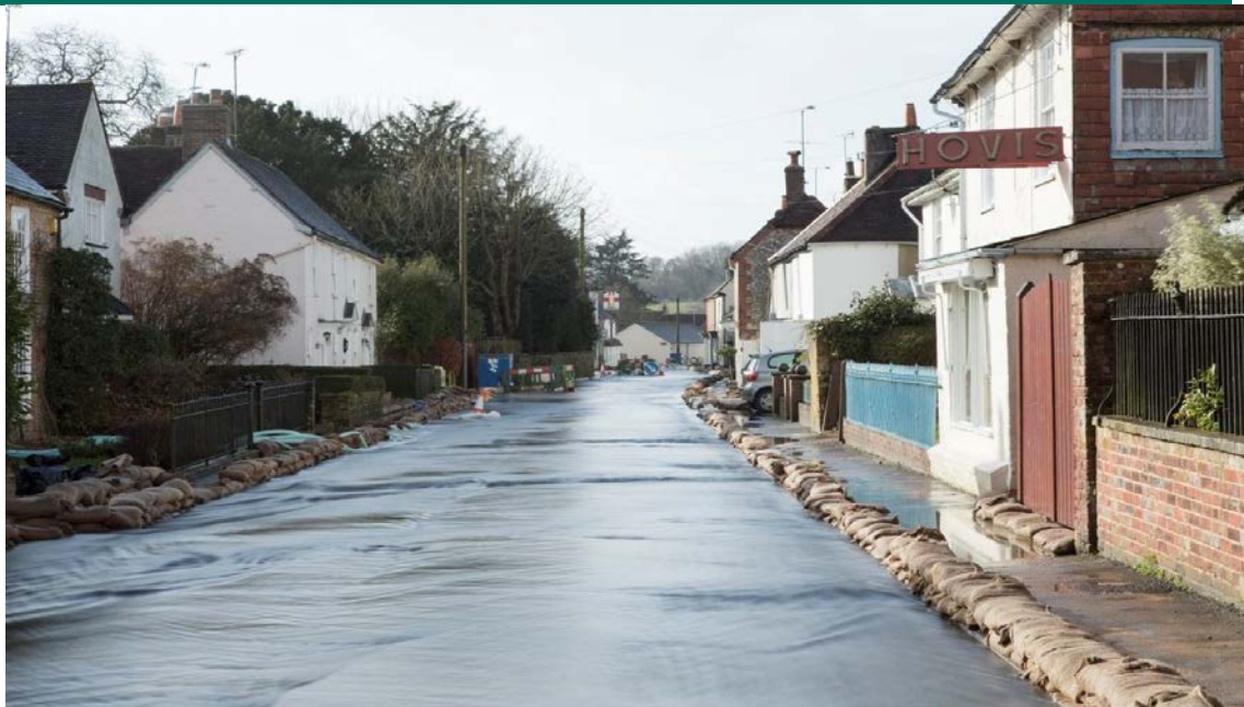
Flood water being confined to the road to protect homes in Hambledon.
