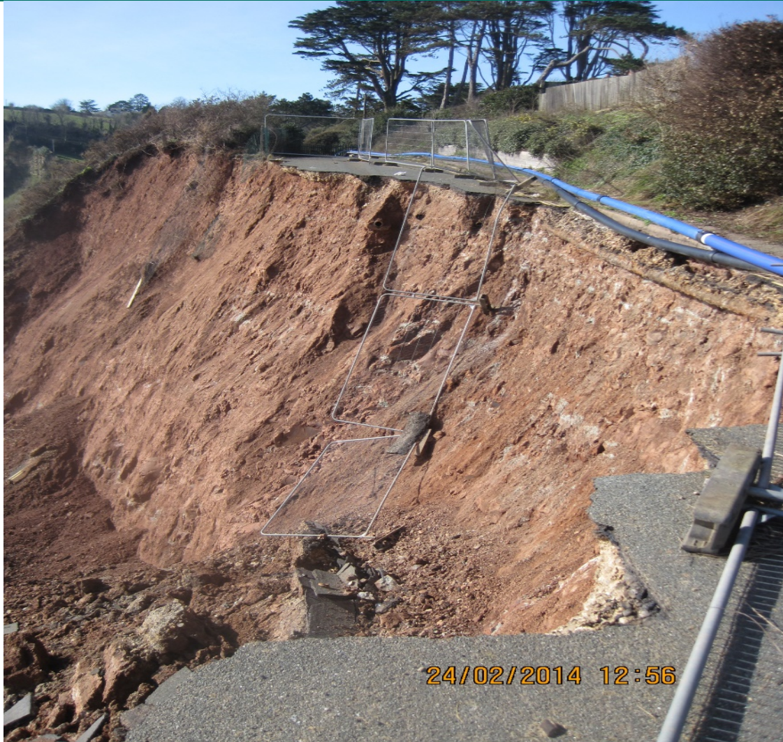
Landslip on local road.
