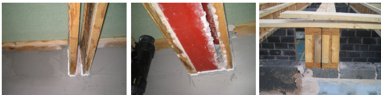
Figure 14 – Multiple adjacent built-in joists and beams
