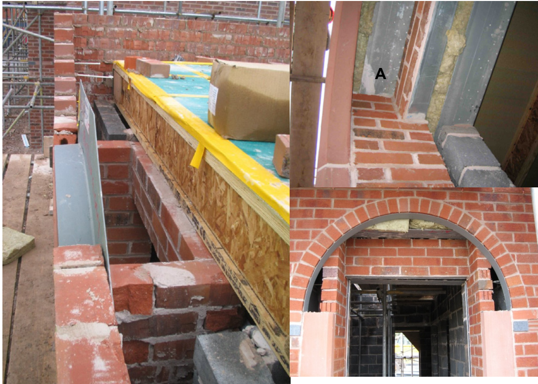
Figure 3 – Construction of recessed front door
