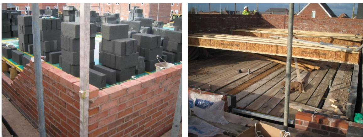
Figure 27 - Intermediate floor construction – external leaf built before inner leaf INAPPROPRIATE MATERIAL AND COMPONENT SELECTION
