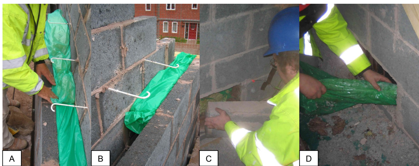
Figure 39 – Horizontal cavity sock being inserted into party wall cavity during construction (A,B) and then being removed again halfway through the coheating test (C,D)
