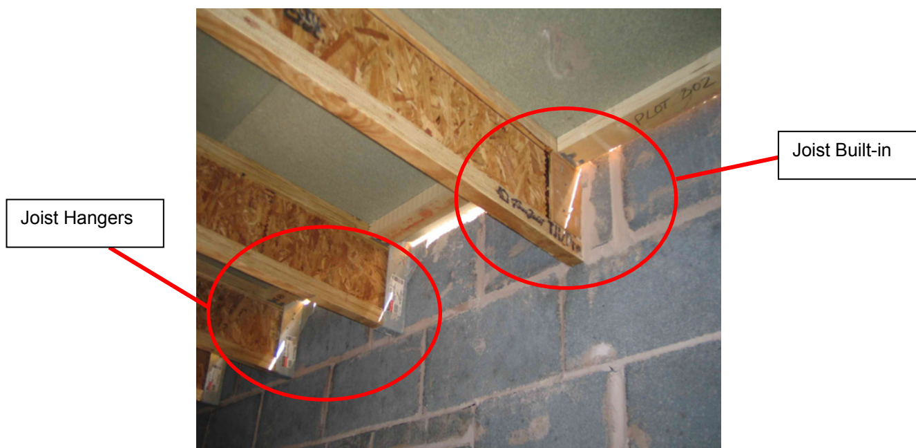
Figure 29 – Intermediate floor built with combination of built-in joists and joists on hangers
