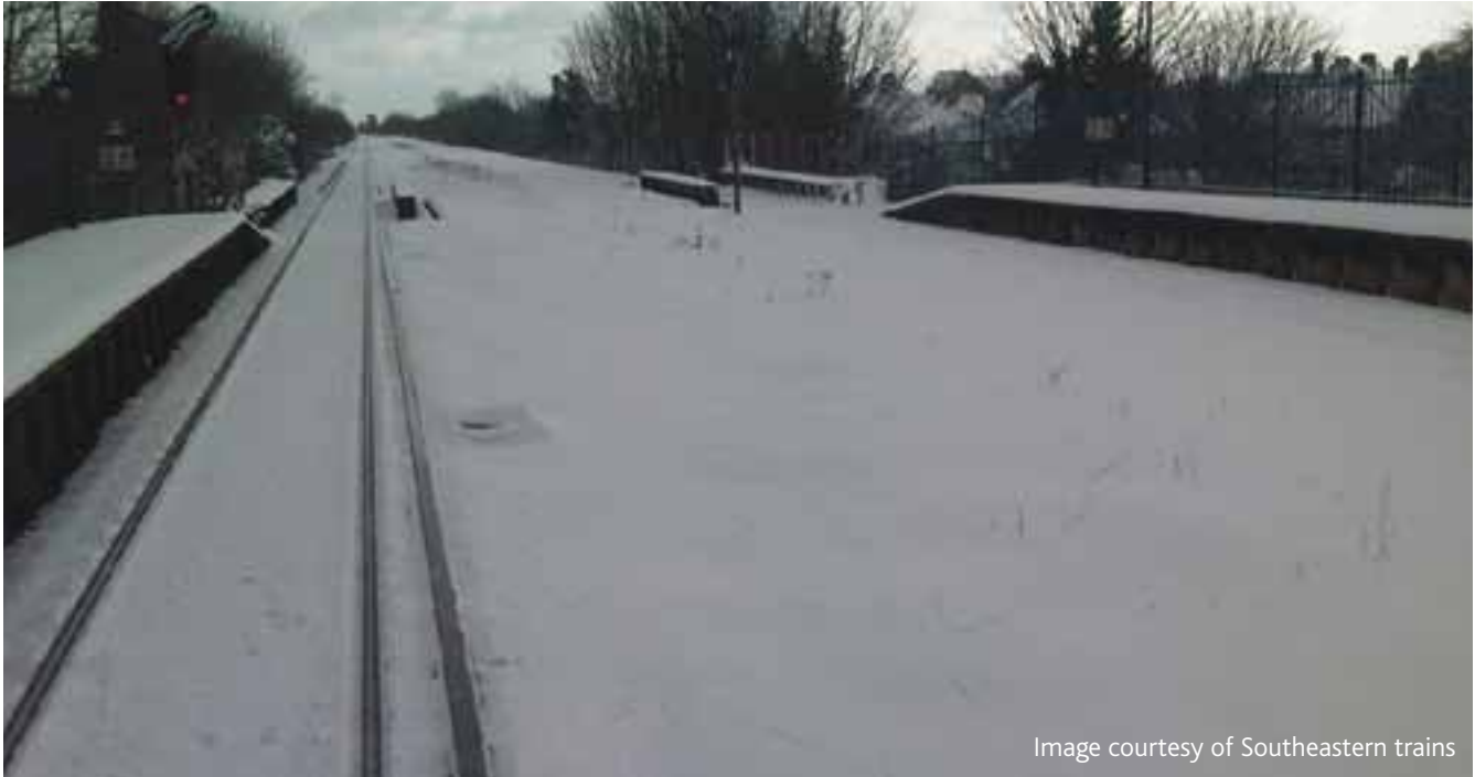
Figure 4.1 Exposed conductor rail in snow
