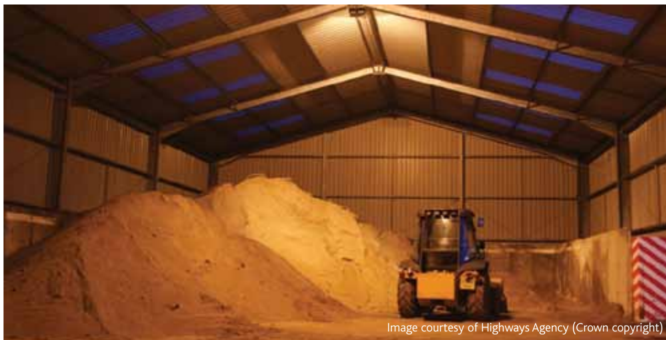
Figure 10.4 – Highways Agency salt barn with loader
