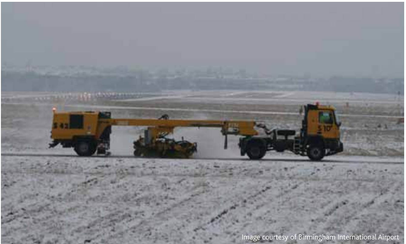
Figure 6.2 Clearing Birmingham International Airport of snow and ice
