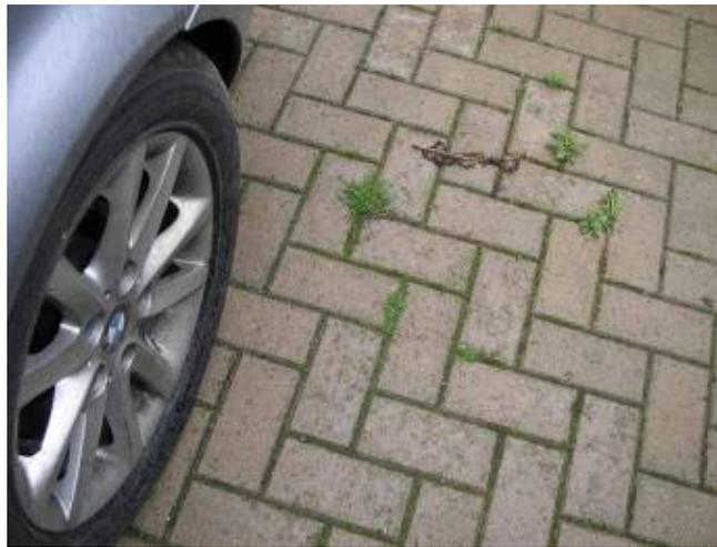
**Figure B1 Concrete block permeable pavement appears clogged**
