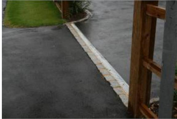
**Figure 2.3 Drainage channel for a driveway**
