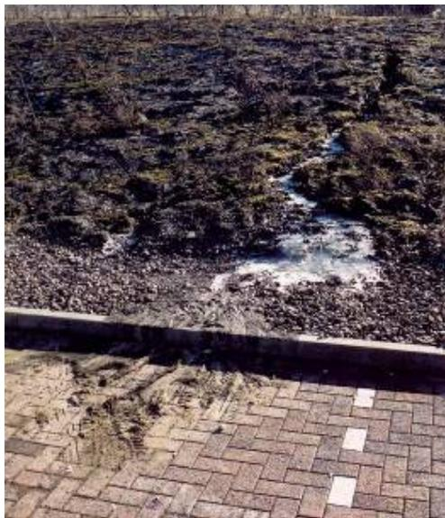
**Figure 2.6 Topsoil washed onto permeable surface**
