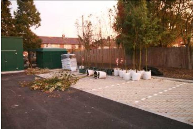
**Figure 2.5 Topsoil spilled onto completed permeable surface**
