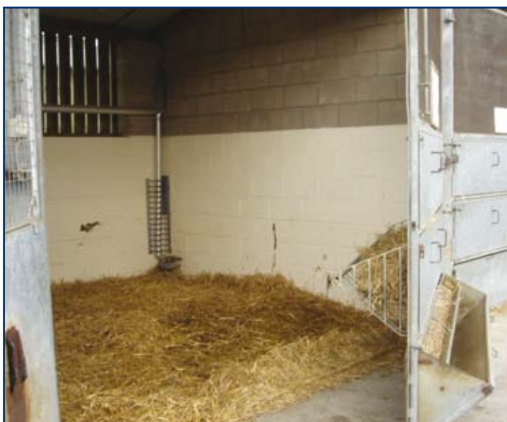
Flexible arrangement of feeding troughs in enclosure door allowing use by cattle, sheep, horse or pigs
